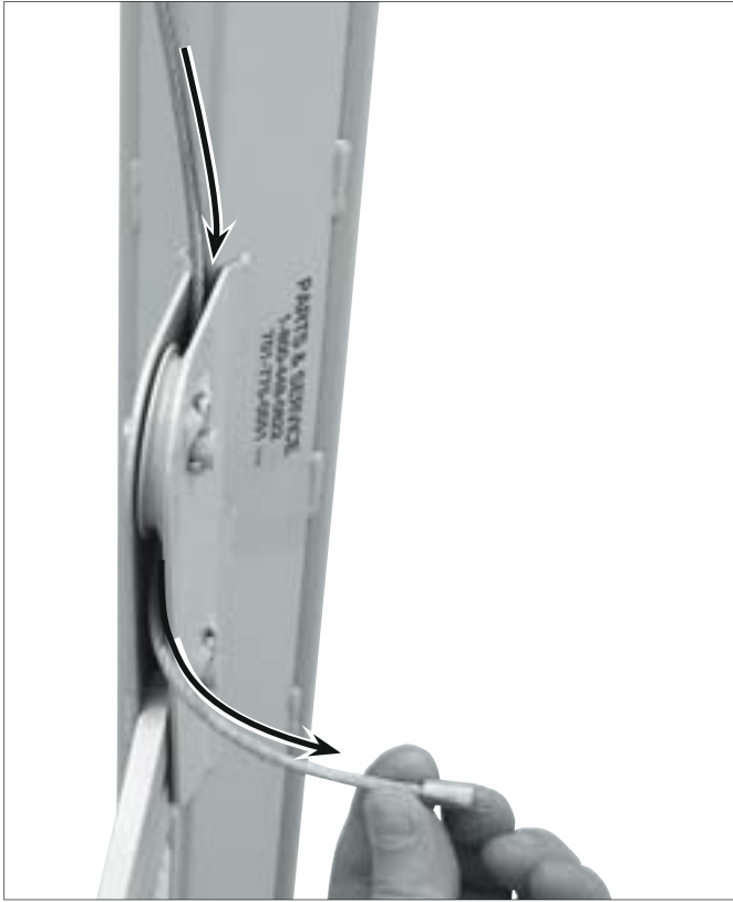
26. Feed the copper crimped end of the cable through the lower frame sheave pocket from the top and out the bottom as shown.
